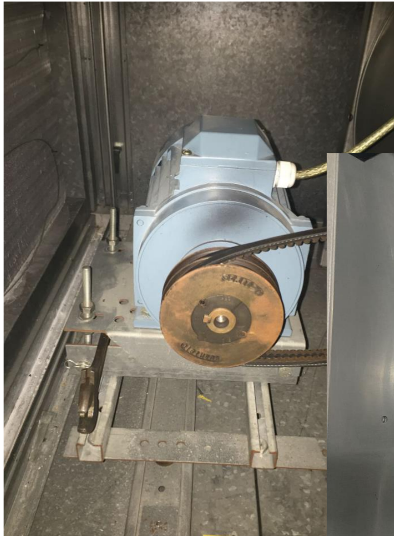
Old belt-driven fans
